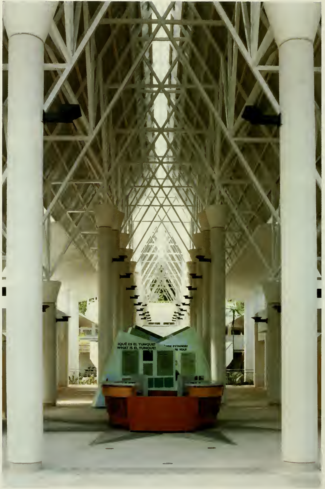
Dominating the central axis is a dramatic roof structure that is at times opaque, translucent, perforated, or skeletal. Photograph: Max Toro
